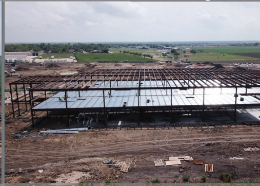
Steel & Decking (Area B) _ 04.26.2023
